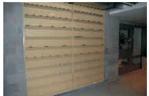
INSTALLED ARCHITECTURAL ACOUSTICAL LOUVERS
